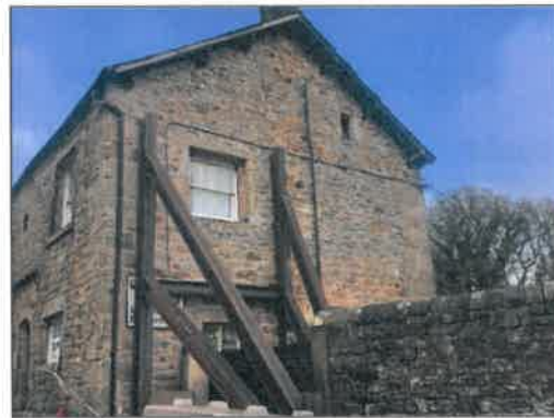
Photo 7: Gable of Section 1.
