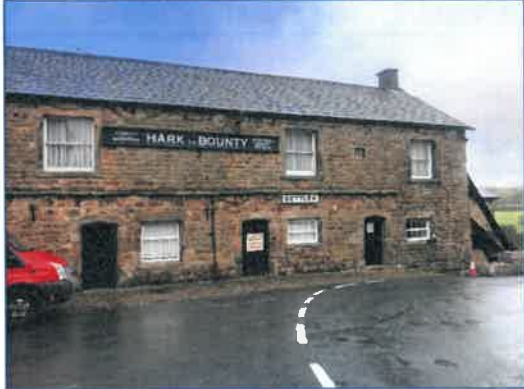
Photo 1: Southern aspect of building.
