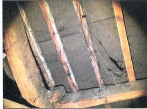
Photo 4: View of liner in Section 1.
