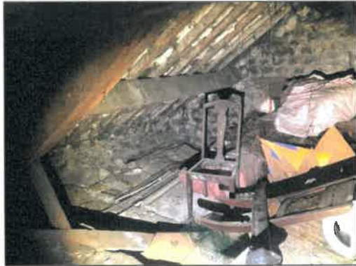
Photo 3: Internal view of void of Section 1.
