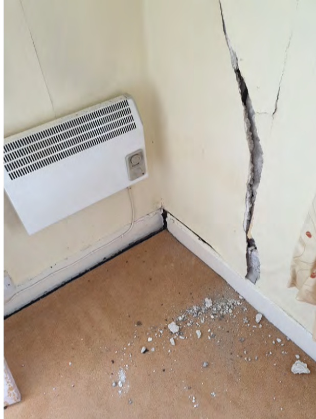
Figure 18 View of damage to floor structure
