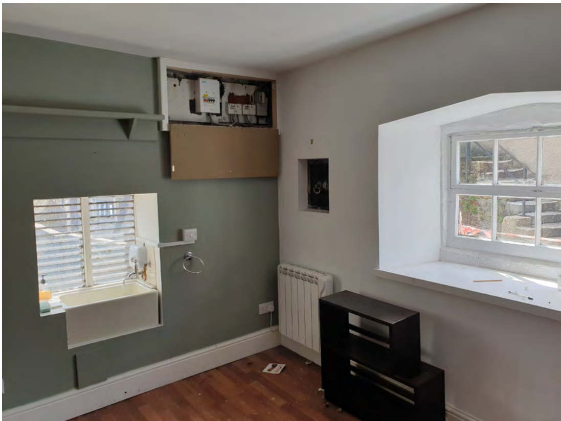
Figure 20 Ground-floor south-eastern room interior
