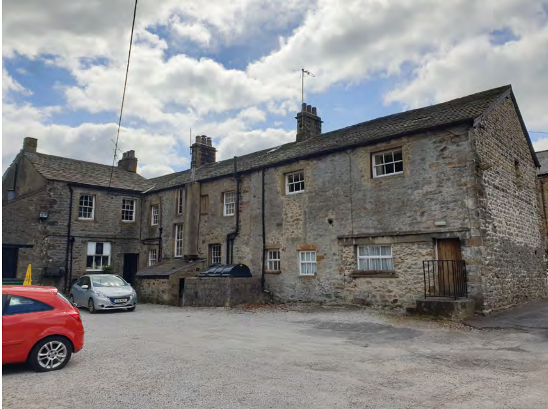
Figure 12 View of rear north-facing façade, looking south-east
