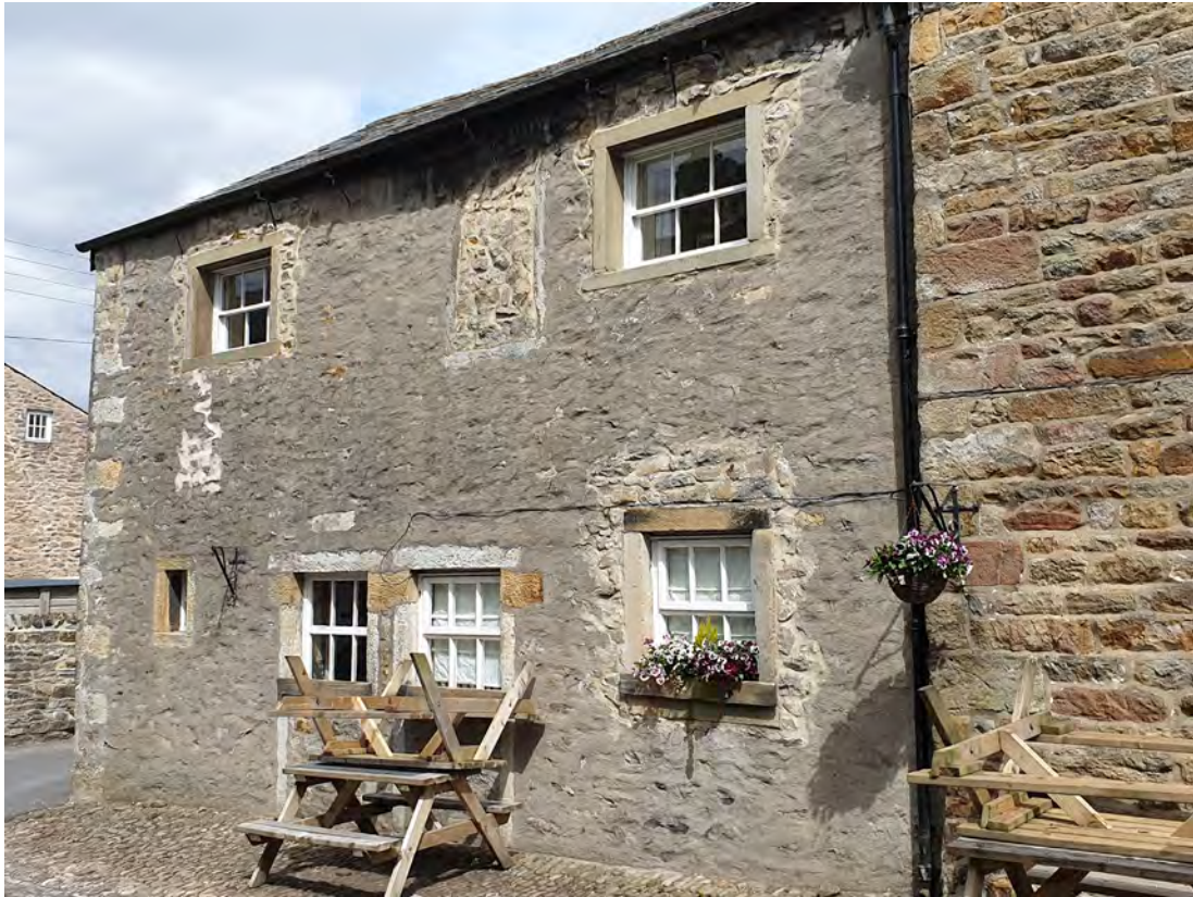
Figure 7 View of converted stables
