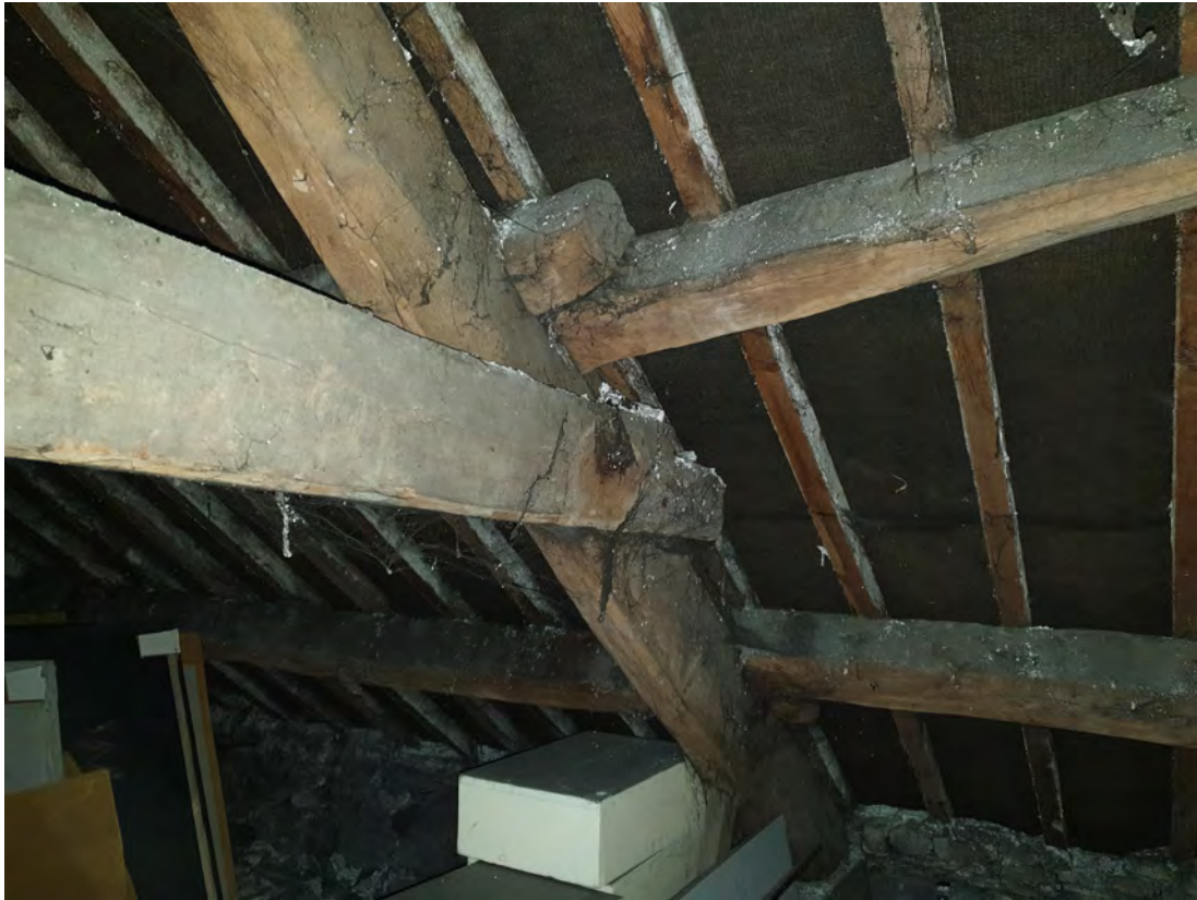
Figure 23 View of roof structure
