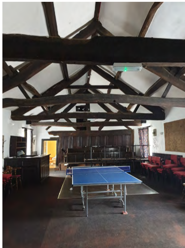
Figure 14 View of large first-floor space with exposed timber trusses
