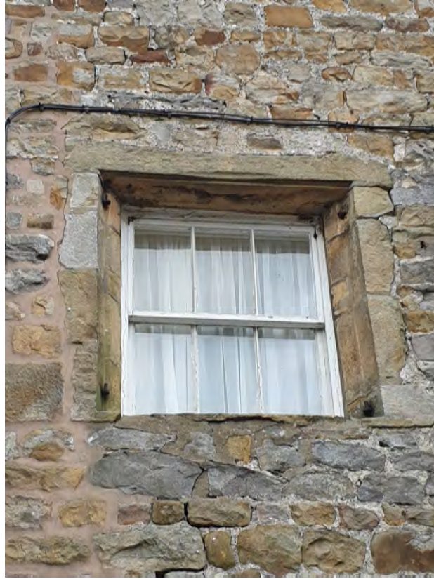
Figure 11 Recessed chamfered window at first-floor level
