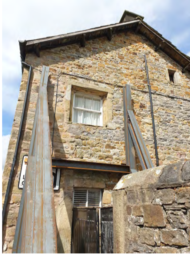
Figure 9 View of east-facing gable elevation, note steel supports
