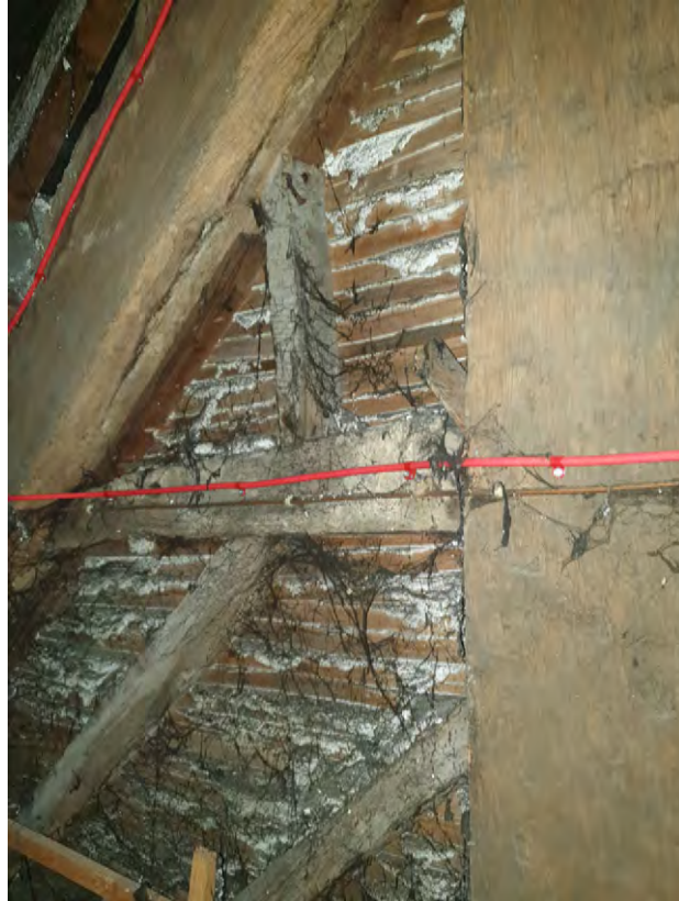
Figure 22 View of surviving lath and plaster
