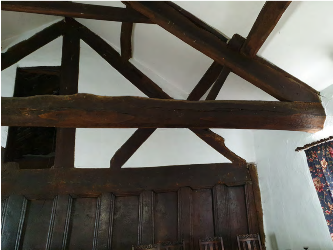
Figure 15 Exposed timber truss detailing
