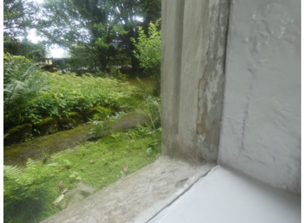
IMAGE 013 – GLASS LINE TO GROUND FLOOR WINDOW
