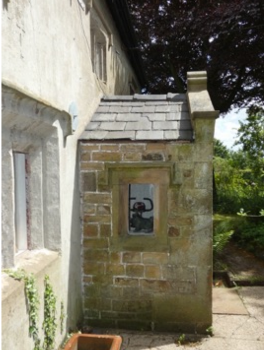
IMAGE 04 – PORCH FIXED LIGHT WINDOW
