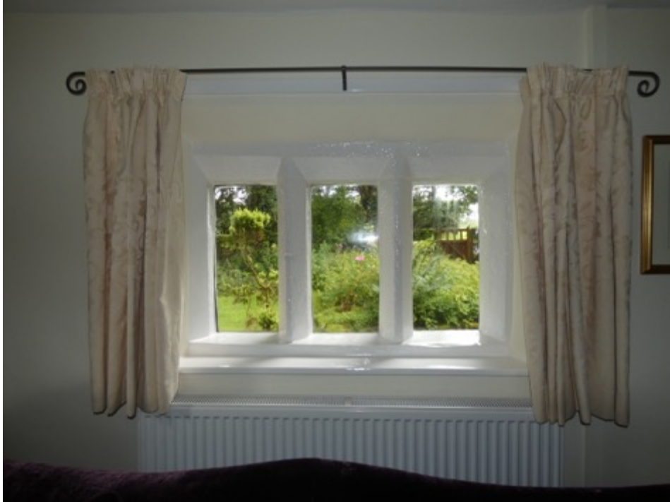
IMAGE 012 – GROUND FLOOR WINDOW, INTERNALLY
