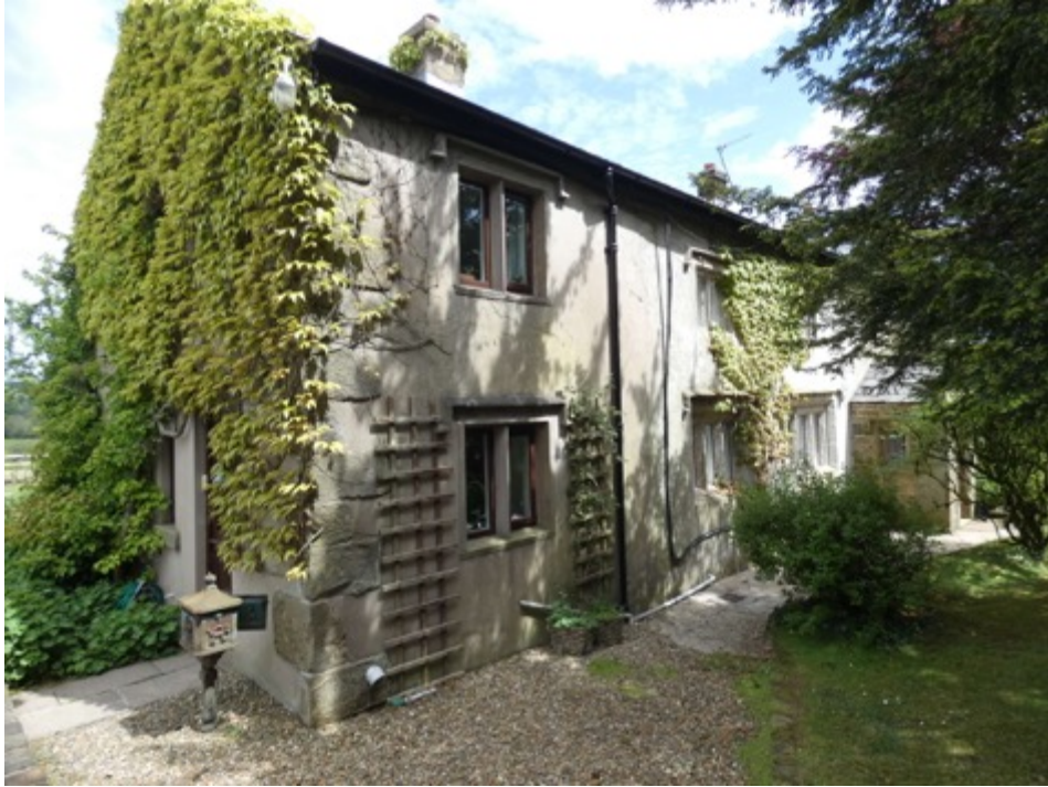
IMAGE 06 – SOUTH ELEVATION, VIEWED FROM SOUTH WEST
