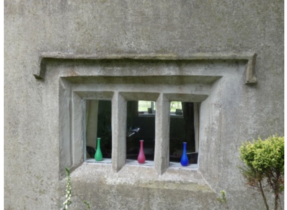
IMAGE 03 – GROUND FLOOR FIXED LIGHT WINDOW
