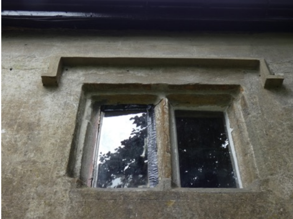
IMAGE 02 – FIRST FLOOR WINDOW WITH OPENING LIGHT
