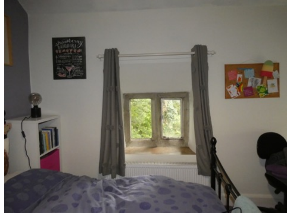
IMAGE 07 – FIRST FLOOR WINDOW, VIEWED INTERNALLY
