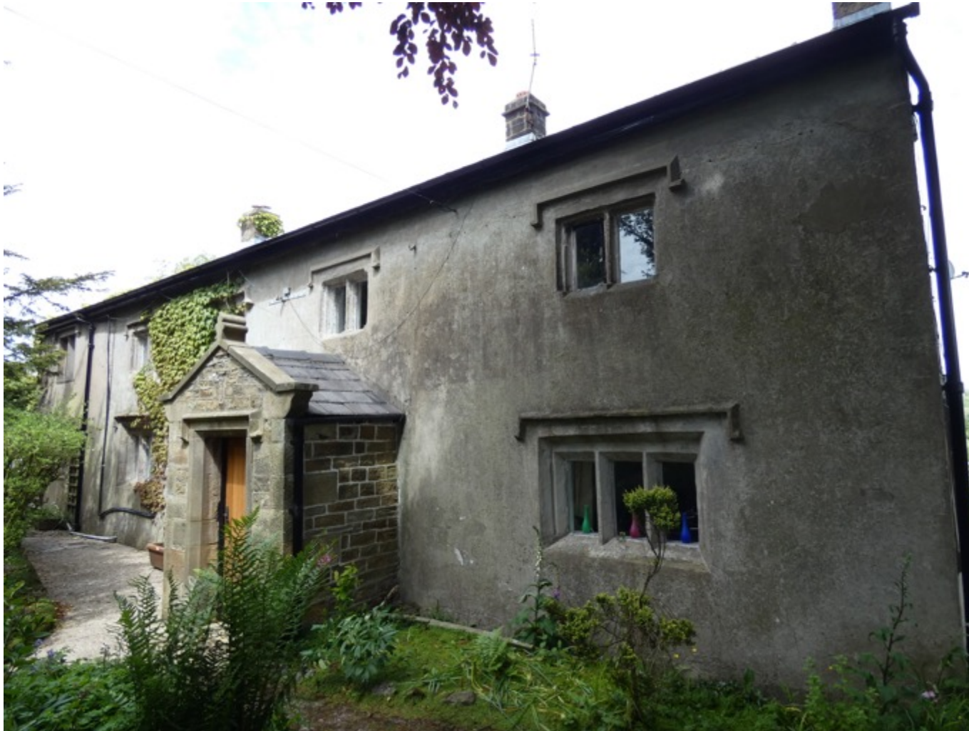
IMAGE 01 – SOUTH ELEVATION, VIEWED FROM SOUTH EAST
