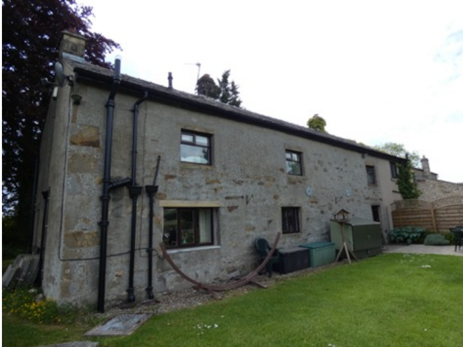
IMAGE 015 – UPVC RAINWATER GOODS TO NORTH ELEVATION
