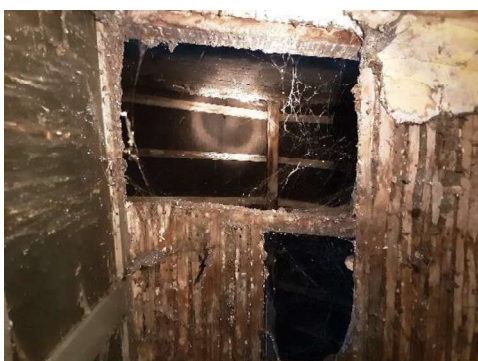
Figure 7: Gap within ceiling of third storey, through which the lined roof is visible.
