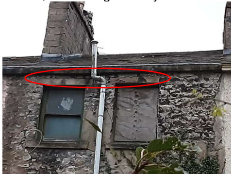
Figure 4: Collection of crevices within the brickwork (circled) and boarded up window on north-western elevation.
