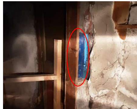
Figure 5: Gap adjacent to the rear doorway (circled).
