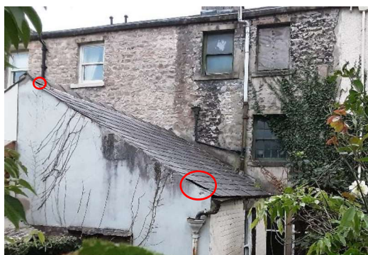
Figure 6: Location of missing tile and area of missing mortar beneath ridge tile on rear extension (circled).
