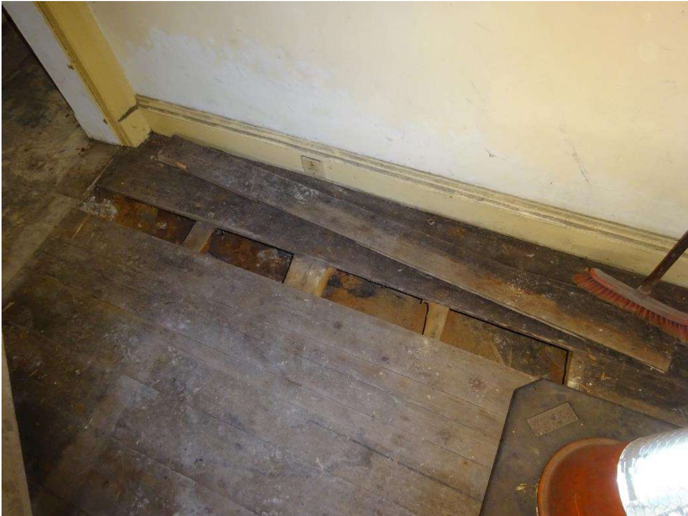
Front Room – Rotten floor joists
