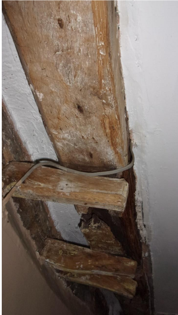
PHOTO 5 – Wedges supporting Timber Beam in Dining Room
