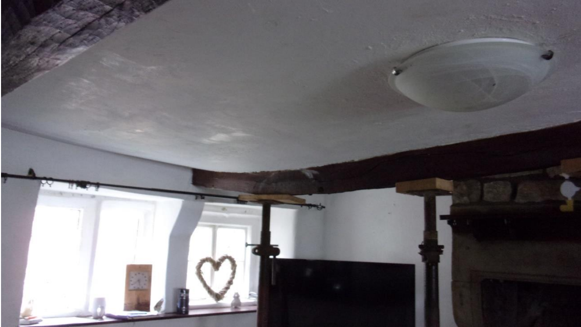
PHOTO 1 – Temporary Propping to Sitting Room Beam
