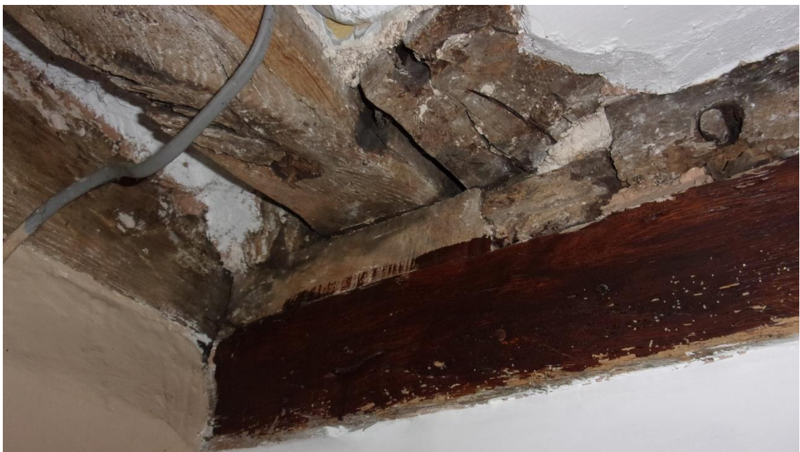
PHOTO 5 – Wedges supporting Timber Beam in Dining Room
