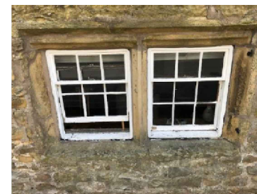
WINDOW 1 Both sash windows
