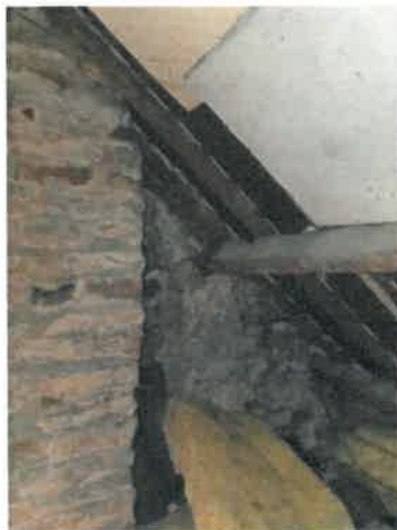
Plate 20: White wooden board over a small section of the roof.
