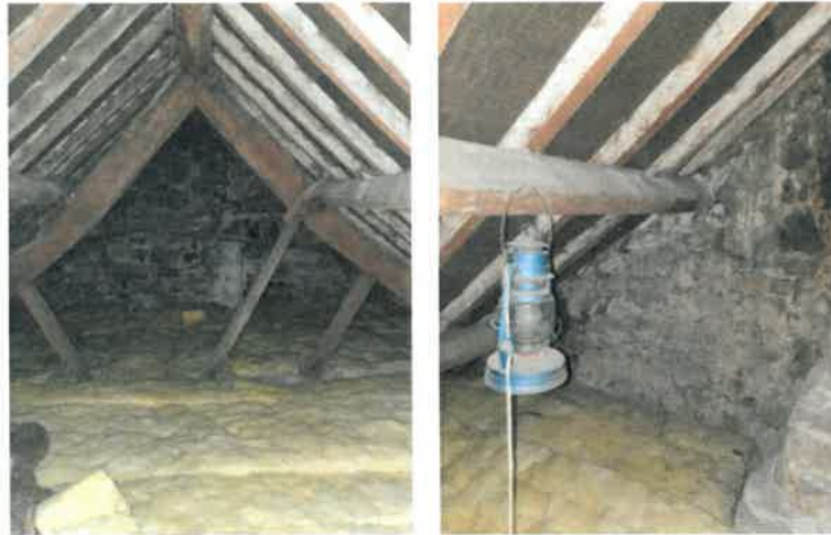
Plates 18 and 19: Gable end and partition wall.
