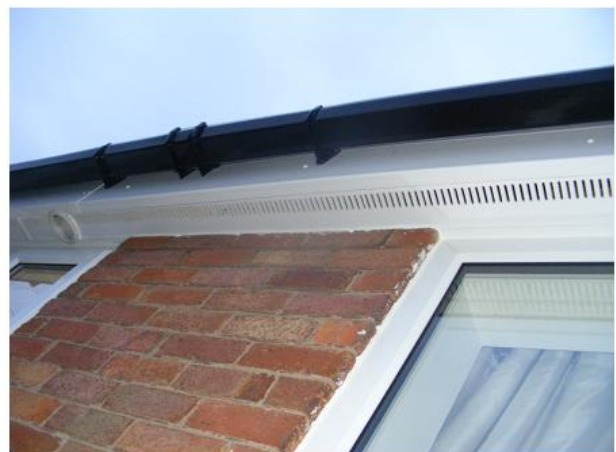
PHOTO 6 Underside of Soffit Box
