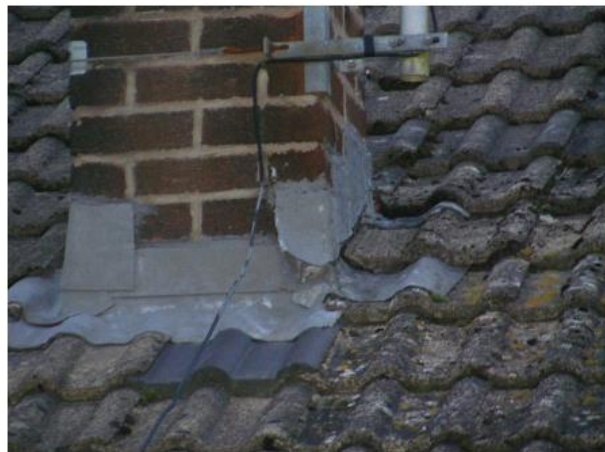
PHOTO 11 Lifted Lead Flashing around Chimney
