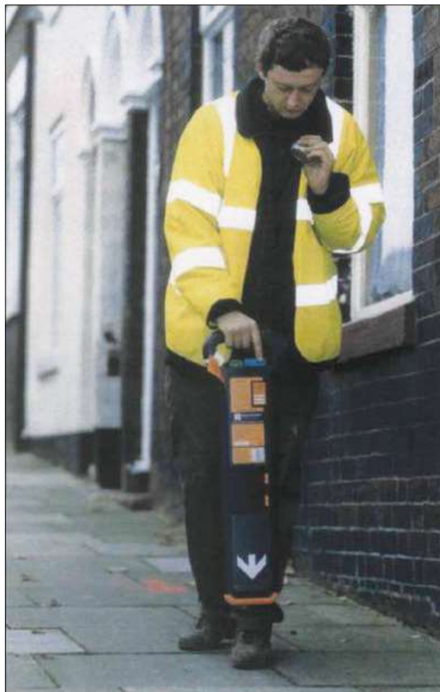
Figure 5 Using a cable locator
