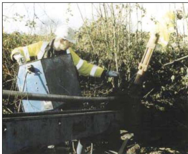
Figure 8 Horizontal drilling being used for laying a cable under a road
