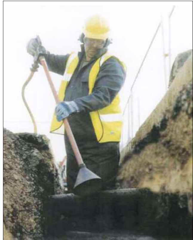
Figure 7 Using an air digging tool
