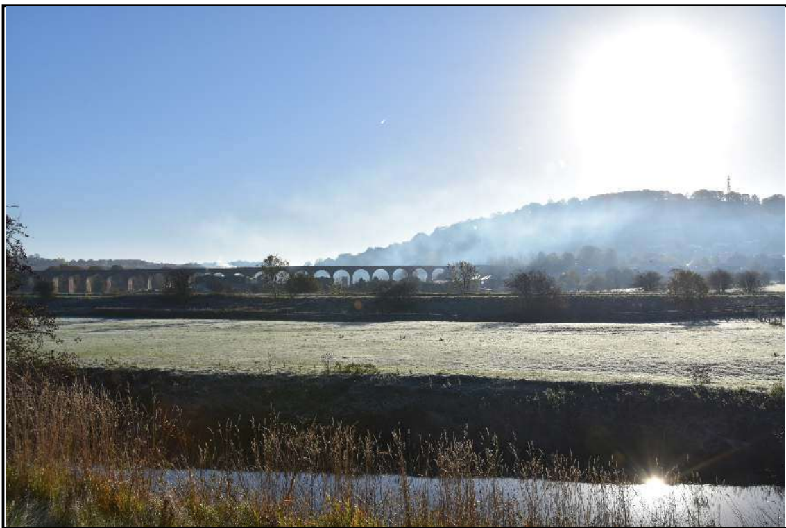
Plate 8 River bank and Whalley Viaduct to the east
