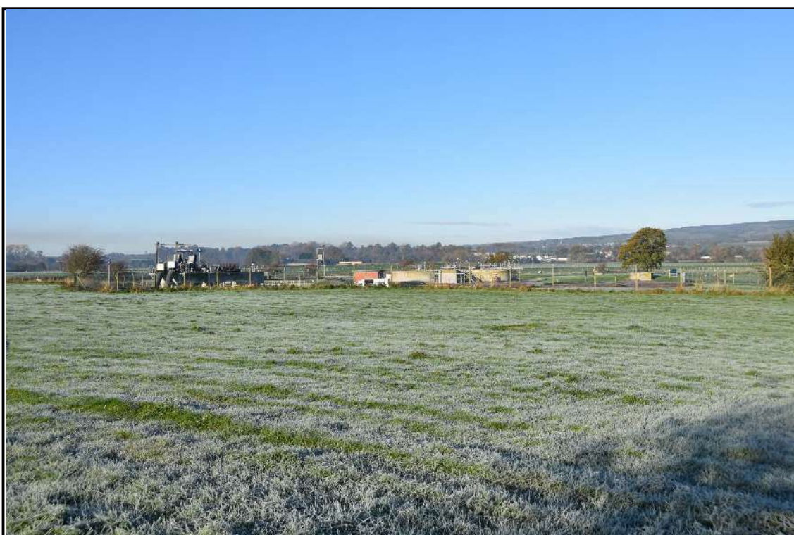
Plate 4 Elevation above the neighbouring sewage works
