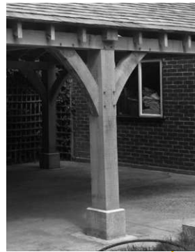
Oak Frame Construction
