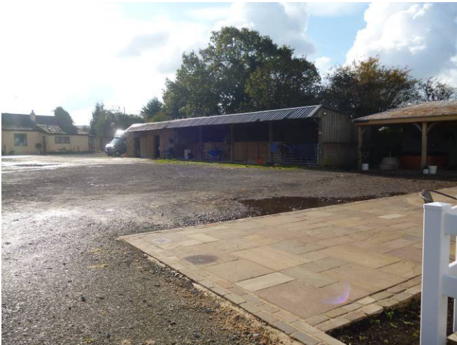
Wooden stable block with negligible bat roost potential.
