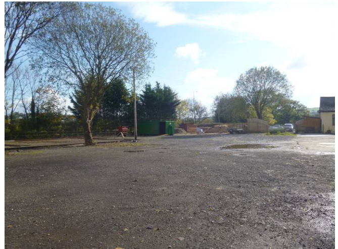
Looking SE across the site.
