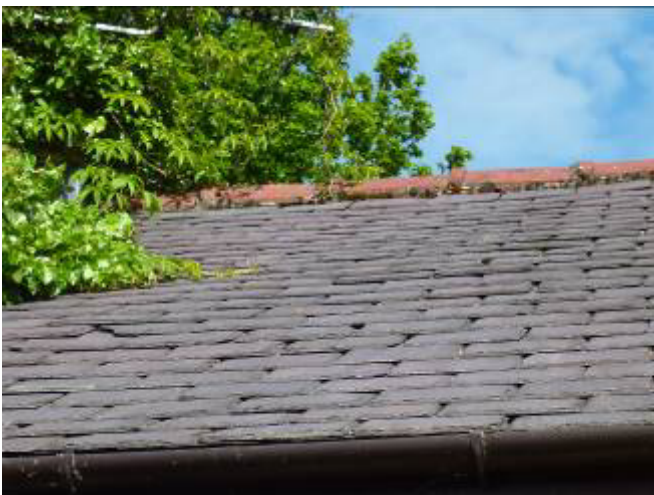
Existing bungalow with negligible bat roost potential. Some localised gaps under ridge tiles requiring supervised removal. Slates generally tight fitting.
