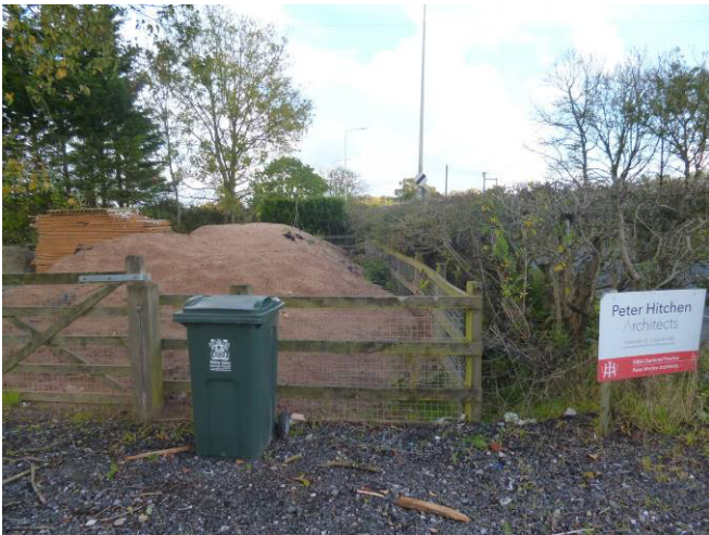
SE corner of site alongside the A59, former ménage area.
