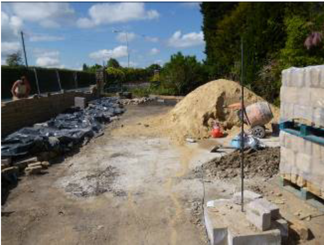
Site frontage with the A59.
