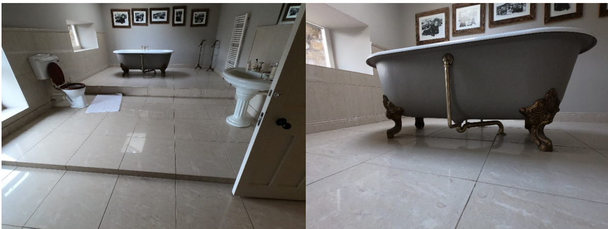
Main bathroom with raised floor to conceal pipework
