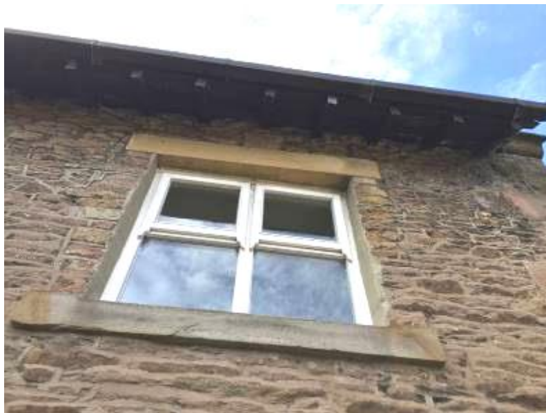
Plate 6: Open eaves on Western elevation
