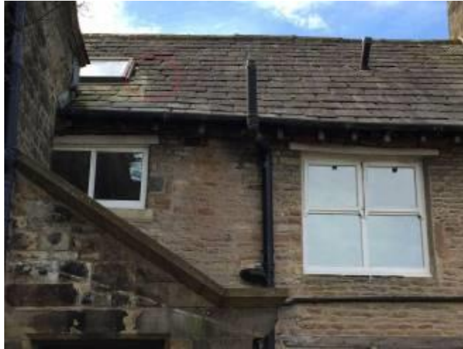
Plate 7: Gaps under tiles indicated
