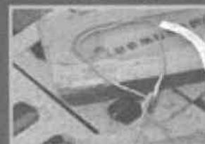
Cavity Wall Tie Repair
