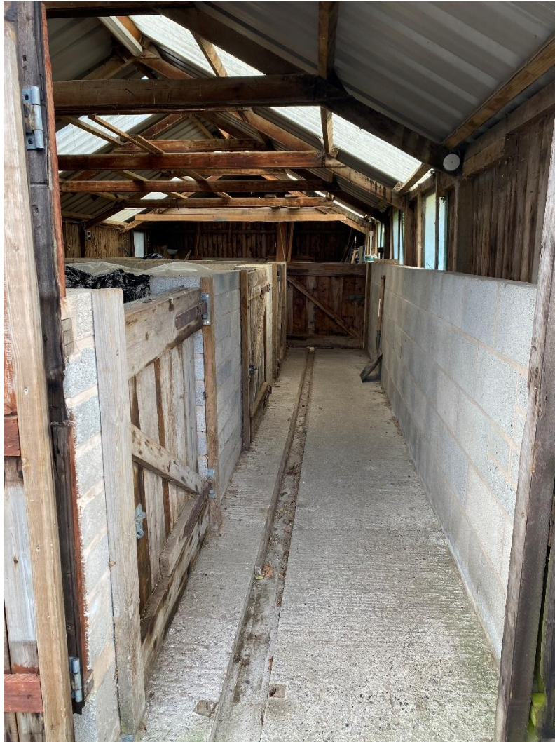
Figure 5 – View at Point E
