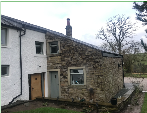
The southeast elevation of the garage extension
