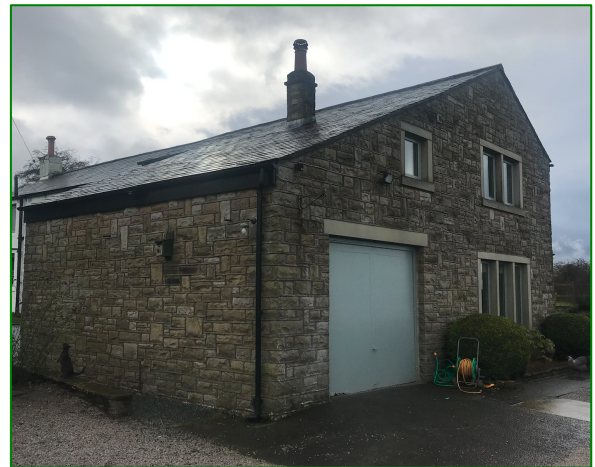
The northeast and northwest elevations of the garage extension
