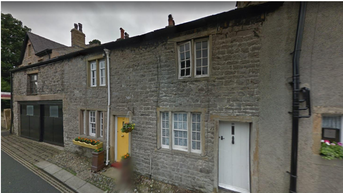
Fig. 2 View of existing garage along the terrace.
