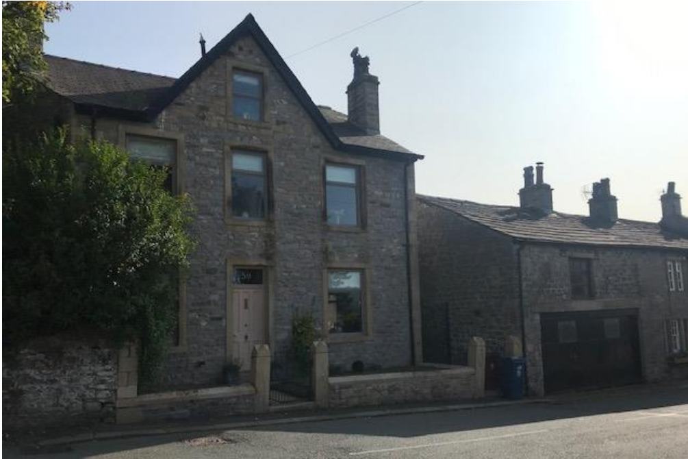
Fig 1: Front (north) elevation of No.59 Downham Road and the adjacent garage
