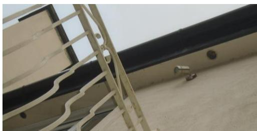
Sitting room outrigger, tiles and flashings very tight fitting, soffits in excellent condition with no possible access points for bats.
