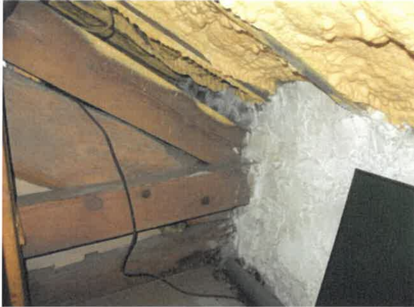
Photo, historic softwood repairs to oak frame and tie beam
