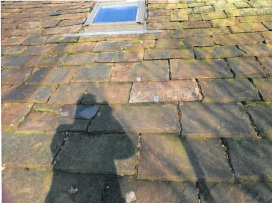
Photo, tabbed and broken stone slates
