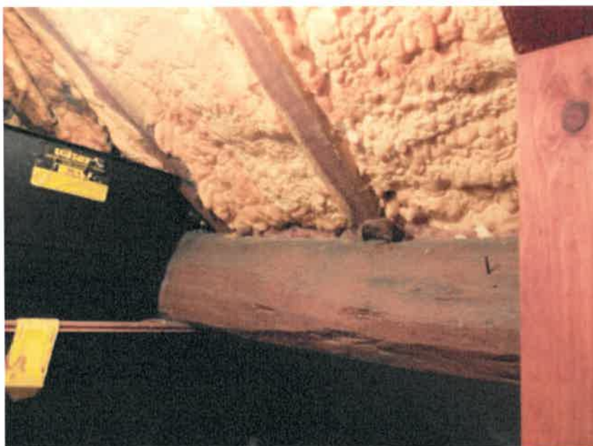
Photo, spray to underside of roof
