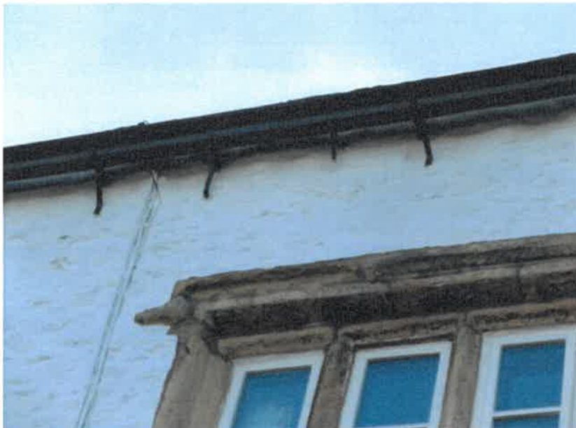
Photo, front ogee gutter
