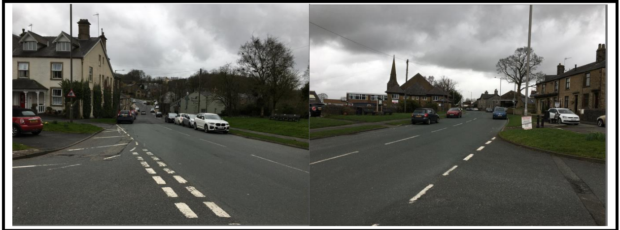
View left and right from Downham Road junction.
