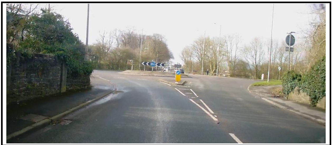
Approach to Pimlico Link Road roundabout from east and west sides
