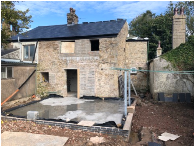
Photo 2: render removed from the rear elevation to reveal patchy stone work which was in a poor state of repair
