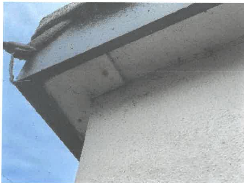
Photo 5: Example close-up of soffit boxes and eaves
