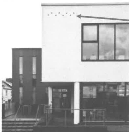
Eight Schwegler Swift Bricks were installed and hidden behind the plastered facade of the new Cullompton Library in Devon
