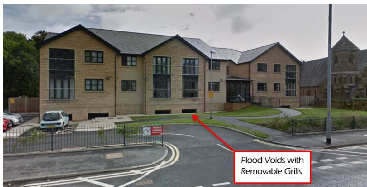
Figure 7.1: Typical Example of Flood Voids
