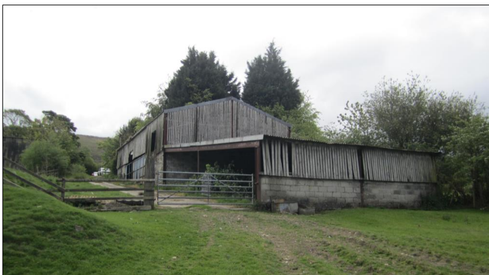
3 Buildings on the lower part of the site to be removed.
