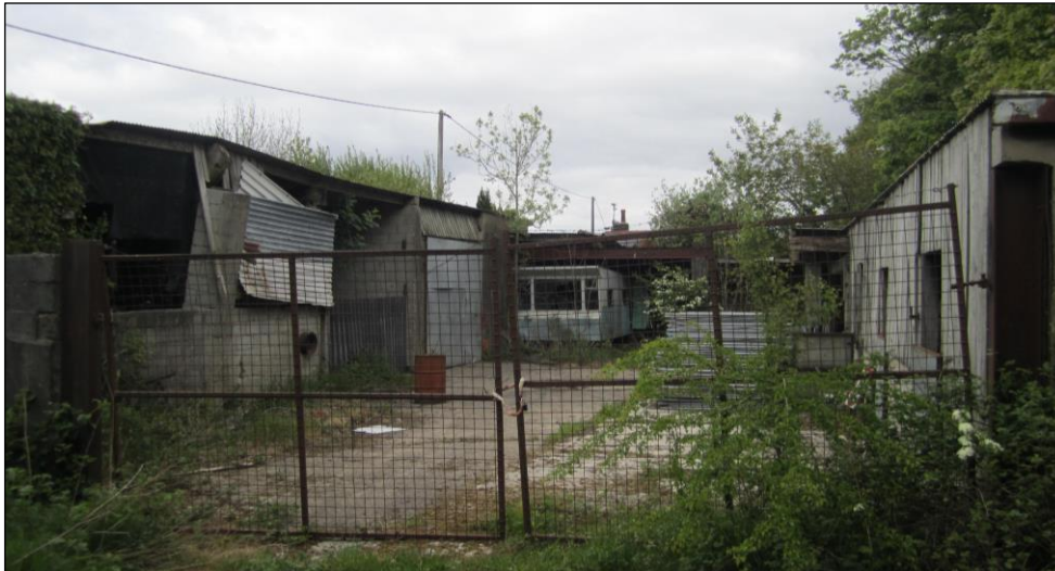
2 Buildings on the upper part of the site to be removed.
