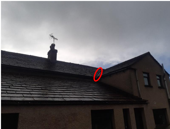
Lead lined valley where two-storey extension abuts to main farmhouse
