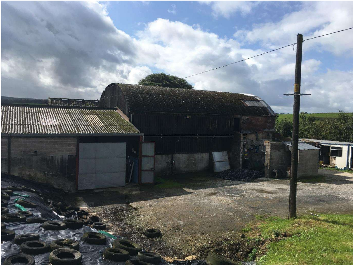
Photograph 2: Dutch Barn viewed from northeast
