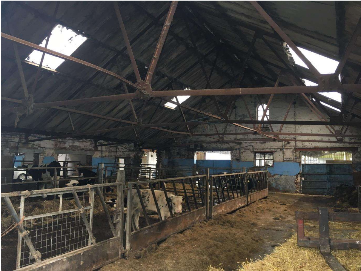
Photograph 4: Internal Rectangular Building
