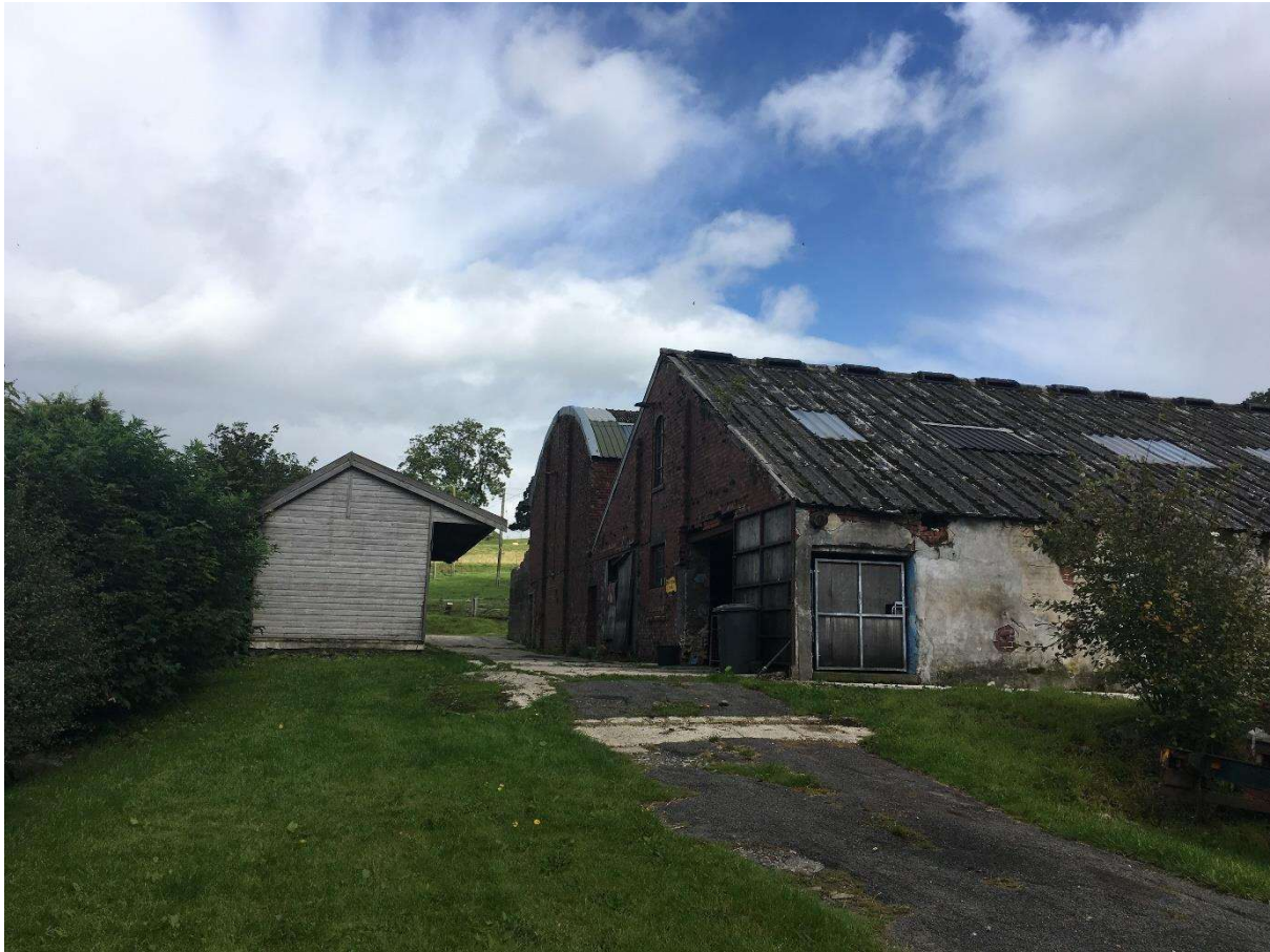
Photograph 1: Proposed buildings viewed from the south
