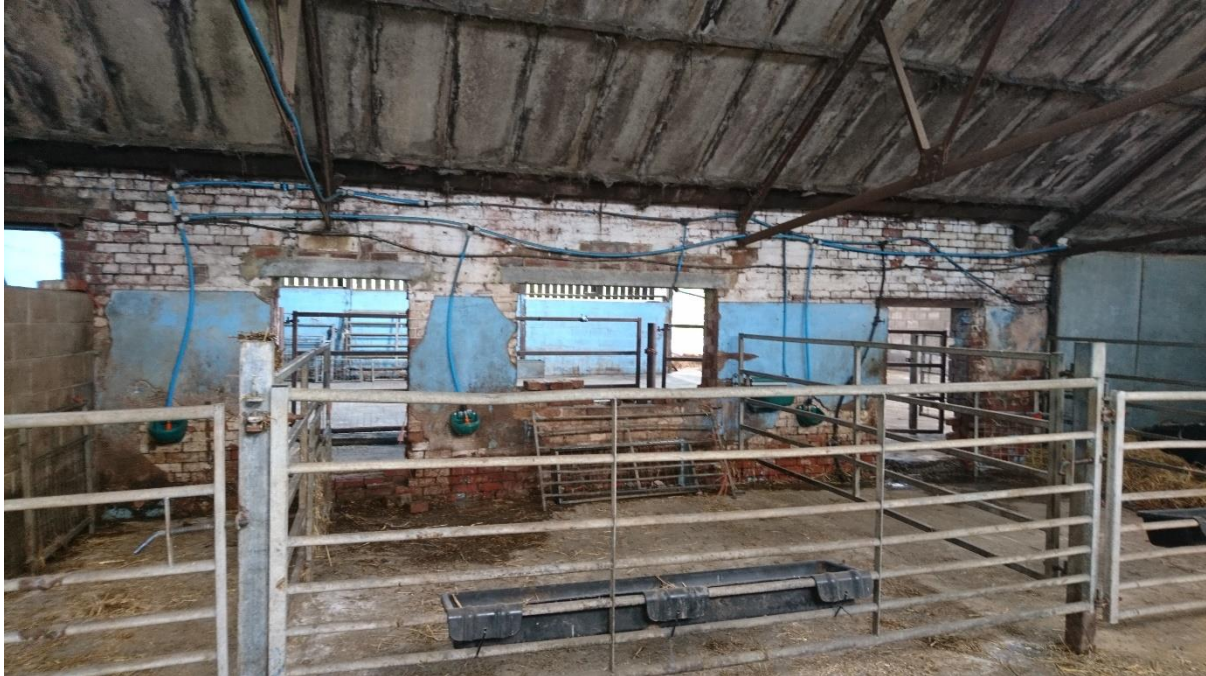
Figure 18: Shared internal wall, punctuated with openings O9 to O15
