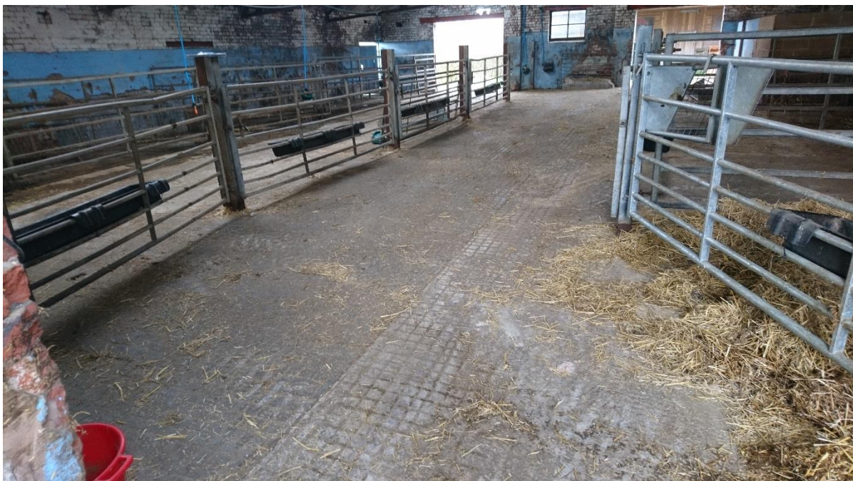
Figure 20: Pitched barn floor
