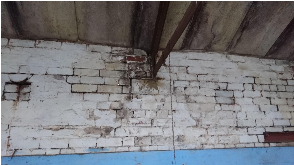
Figure 6: Padstone truss bearings
