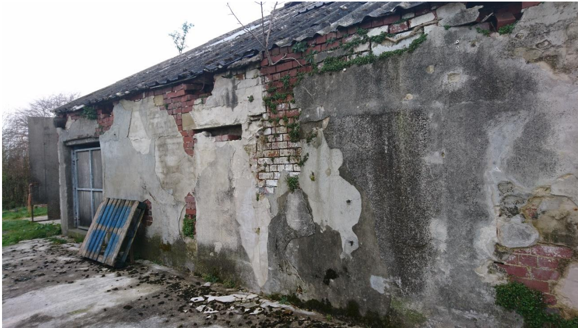
Figure 12: View of the southern elevation, looking west
