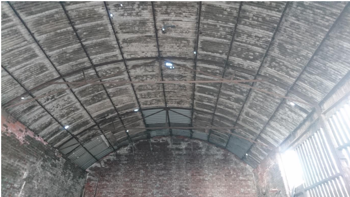
Figure 4: Internal view of the arched roof structure
