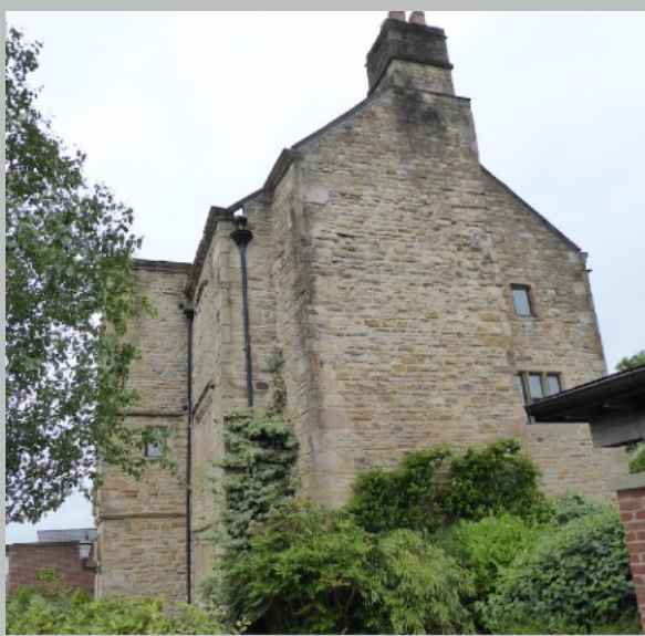
Plate 6. Massive chimney breast on RH (E) gable
