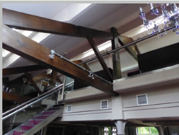
Plate 24. Exposed pine roof truss
