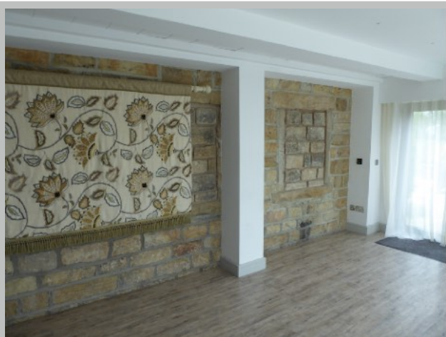
Plate 23. Blocked window openings
