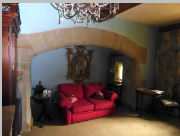
Plate 11. Fireplace with segmental stone arch in (former) kitchen
