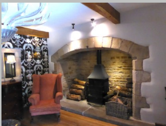
Plate 10. Fireplace with segmental stone arch in (former) middle parlour
