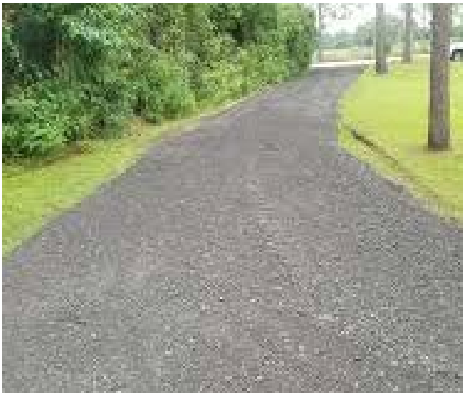
Existing footpath link upgraded. Potential to break up existing bitmac where it remains and top with road planings. Result will be a sustainably sourced pathway with the following benefits: Existing driveway where removed can be crushed and used as surface to footpath meaning material will not have to be taken off or brought on to site.
