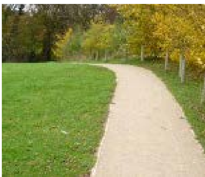
Further informal footpaths are proposed linking the PROW with the main hotel car park and additional bedroom spaces. These routes take advantage of the existing tree cover and would take the line of least resistance through the trees. Surface to be breedon gravel or similar.
