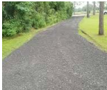
Existing footpath link upgraded. Potential to break up existing bitmac where it remains and top with road planing. Result will be a sustainability sourced pathway with the following benefits: Existing driveway where removed can be crushed and used as surface for footpath meaning material will not have to be taken off or brought on to site.
