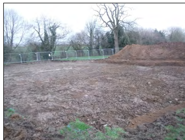
Open area, looking NW.
