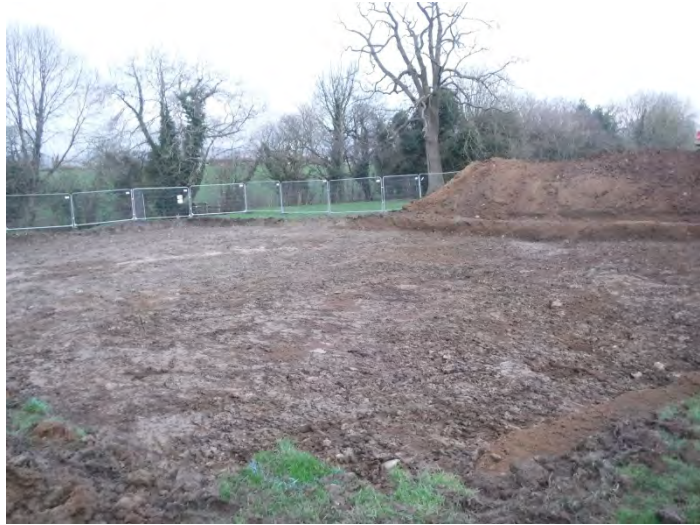
Strip, Map and Record excavation area, looking north-west.
