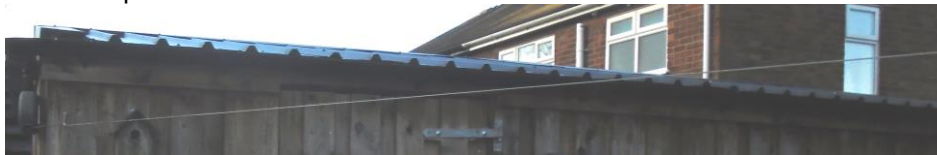
The shed roof has a slight pitch with a corrugated steel sheet roof.
