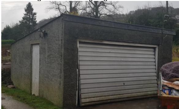
Front west and side north elevations
