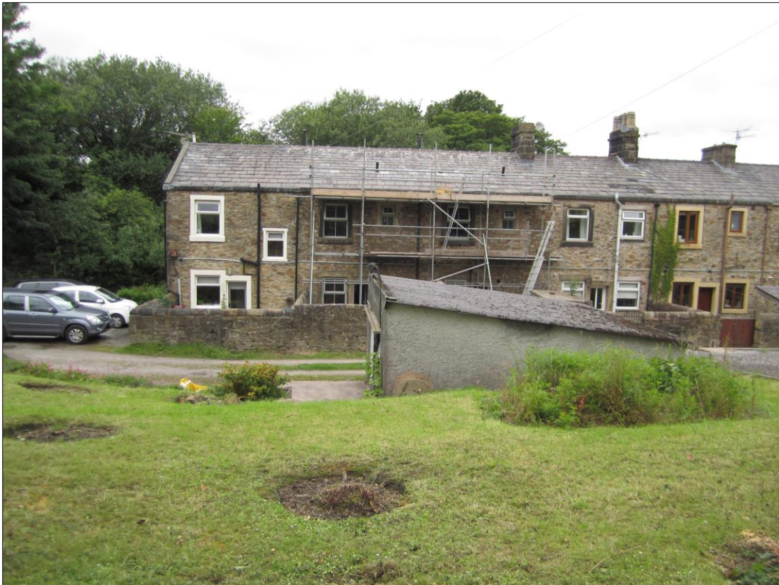
4 View across the site facing north.
