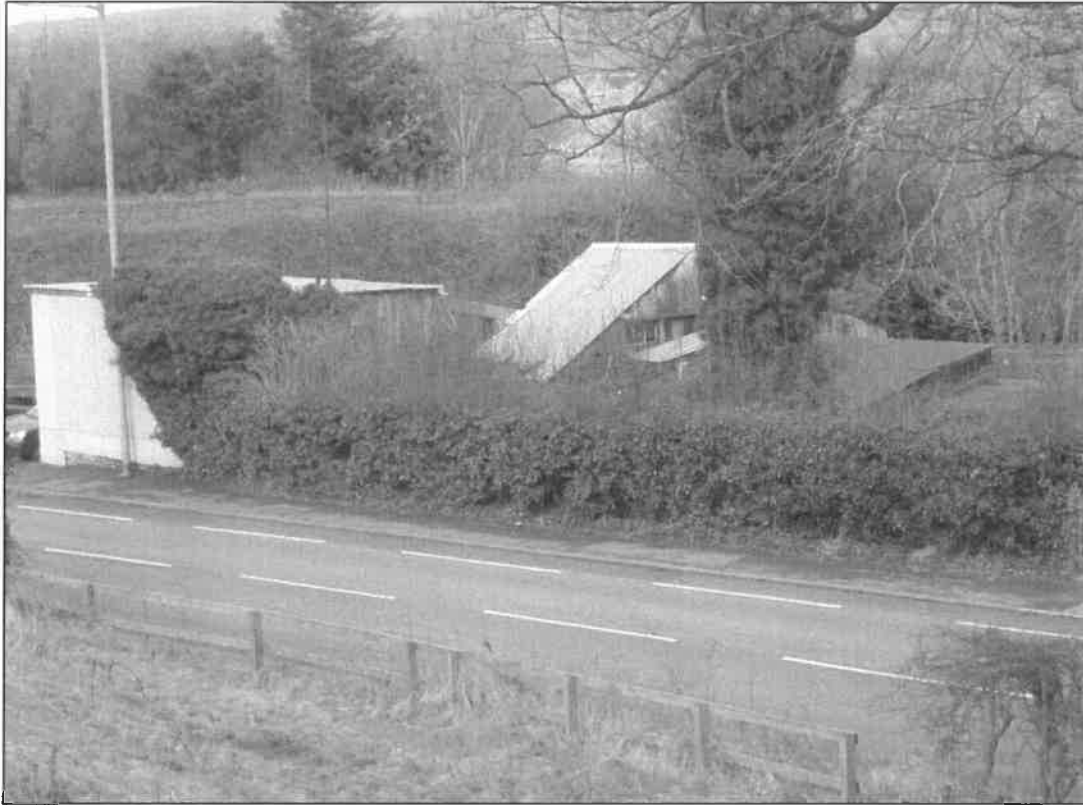
3 The car repair garage adjacent to the west of the site with the railway banking to the rear. Photograph taken from Nab Rise looking north west. .
