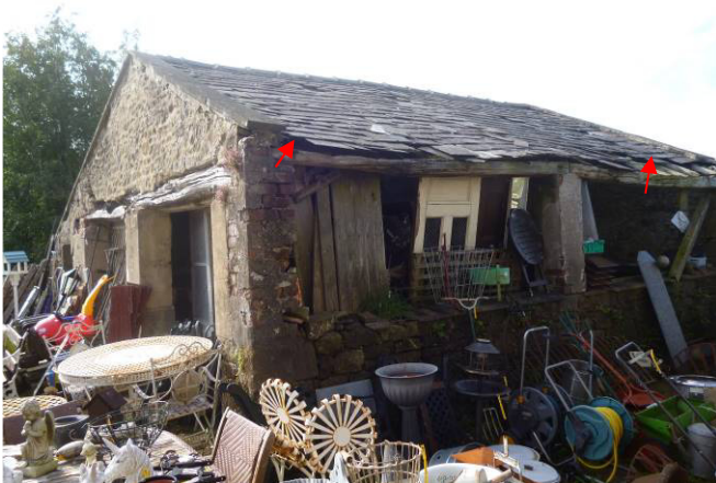
Target Note 1: Outbuilding with multiple potential bat roost features, internal roof with no lining.
