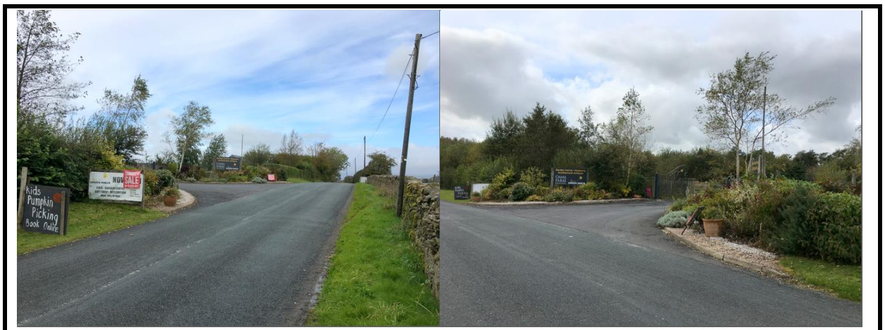
View to access from south and north sides
