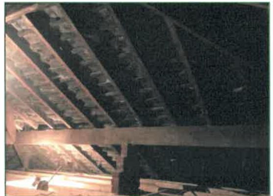
Showing the internal loft void
