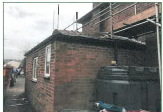
The single-storey extension (to be extended)
