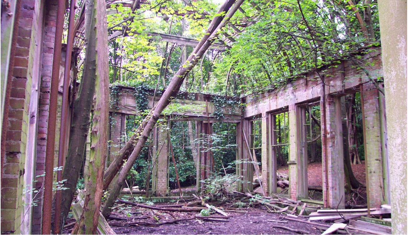
Figure 5) The Orangery interior pre-conversion showing brick piers and concrete lintels
