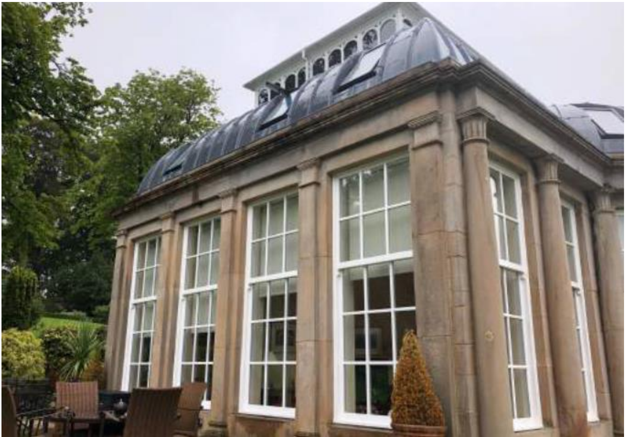
Figure 6) Post-conversion (western elevation)
