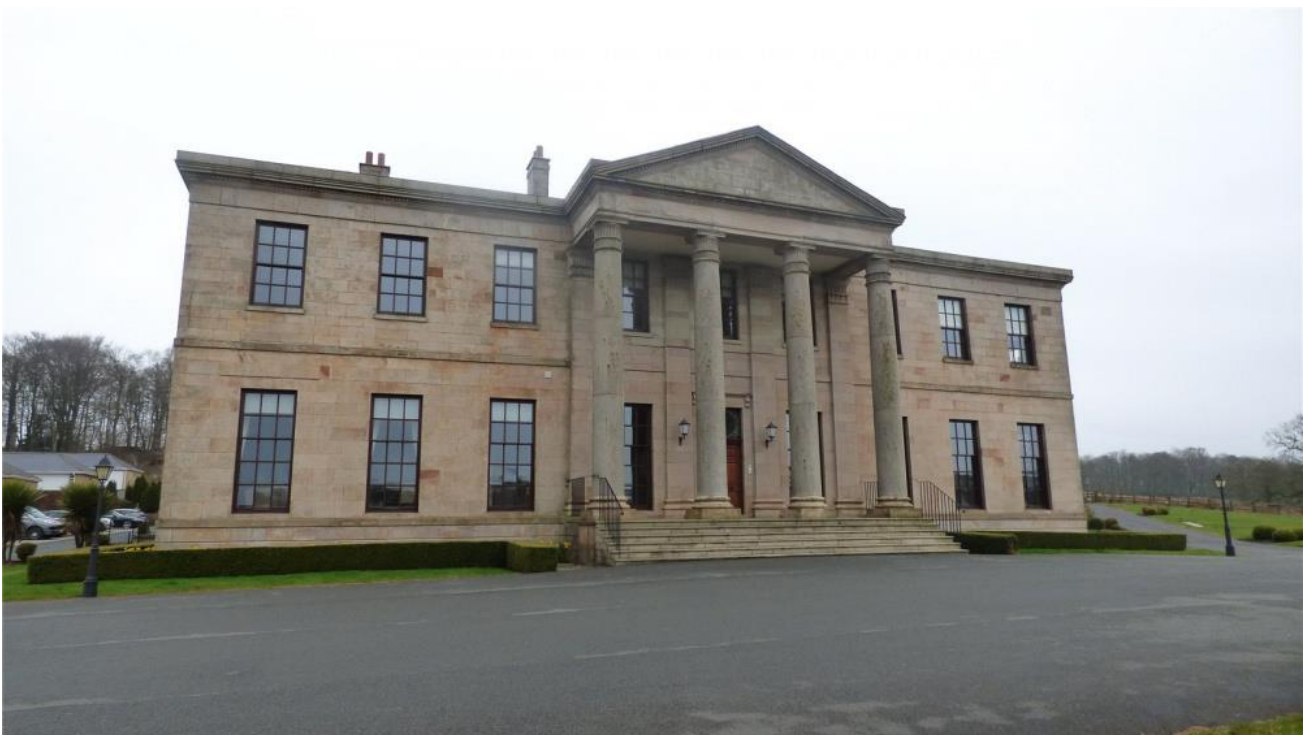
Figure 10) The renovated Hall
