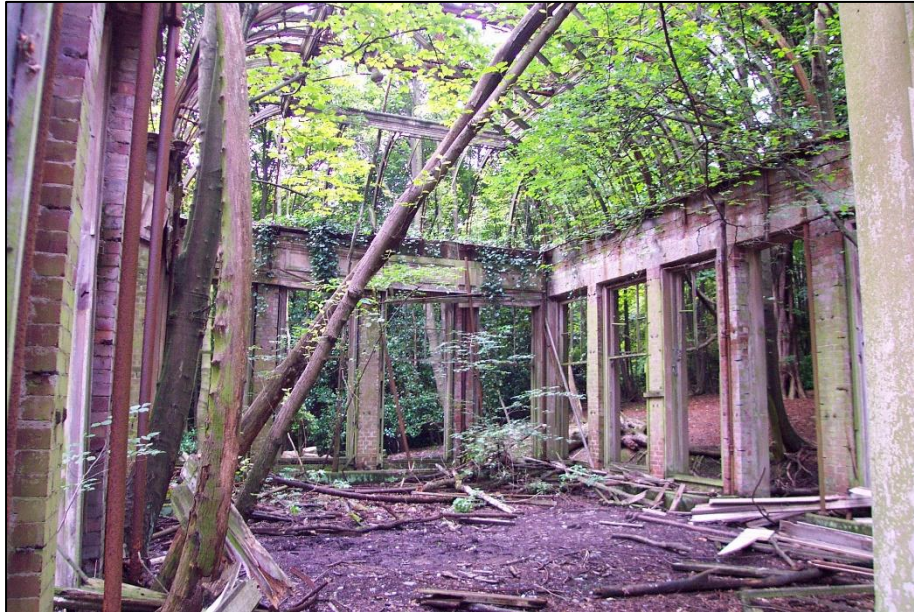
Figure 5. Internal view pre-conversion.
