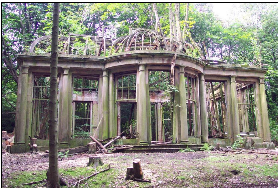
Figure 2. Front elevation pre-conversion.
