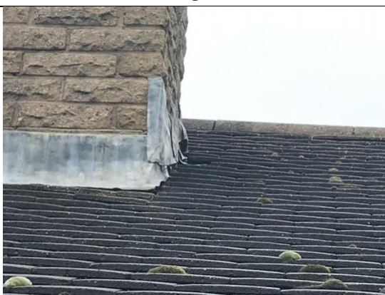
Gaps around lead flashing
