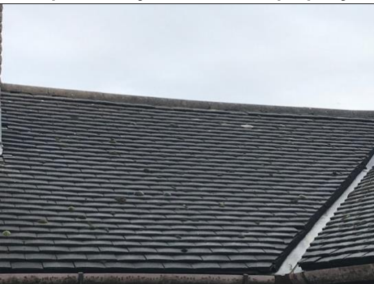
Gaps under tiles near top of roof
