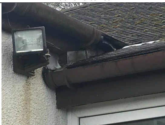
Gaps in roof joints at rear of property
