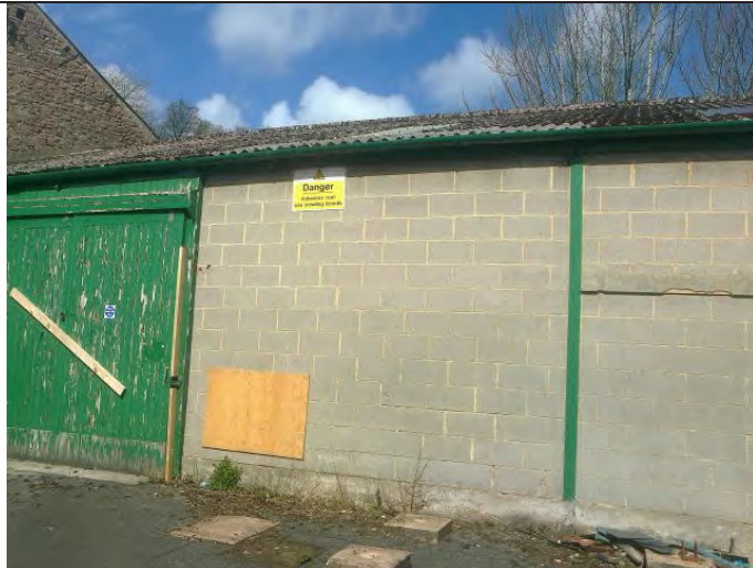
Photograph 7 (facing N): Small buildings adjoining the barn along the northern site boundary with corrugated asbestos roof.
