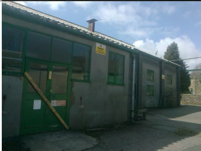
Photograph 9 (facing N): Warehouse building on Area 1.
