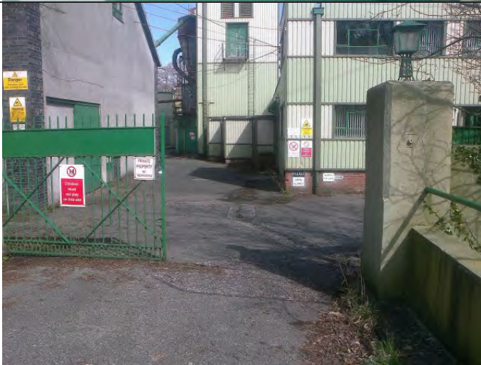
Photograph 5 (facing E): Central portion of Area 1 showing the timber store (left) and office building / warehouse (right).
