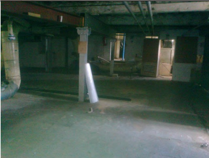
Photograph 3: Inside mill building showing thick concrete floors.
