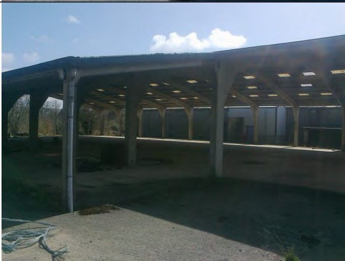
Photograph 12 (facing NW): Open sided timber store to the south of Area 1.
