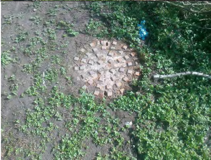
Photograph 29: Drain noted onsite.
