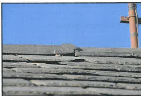
Image slate roof coverings (lhs) and image showing example gaps between slate at the ridge (rhs)
