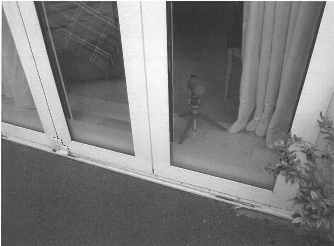
1. Opaque glass obscuring the difference in height between the timber floor on the inside and the tarmac drive on the outside 32 Copperfield Close.
