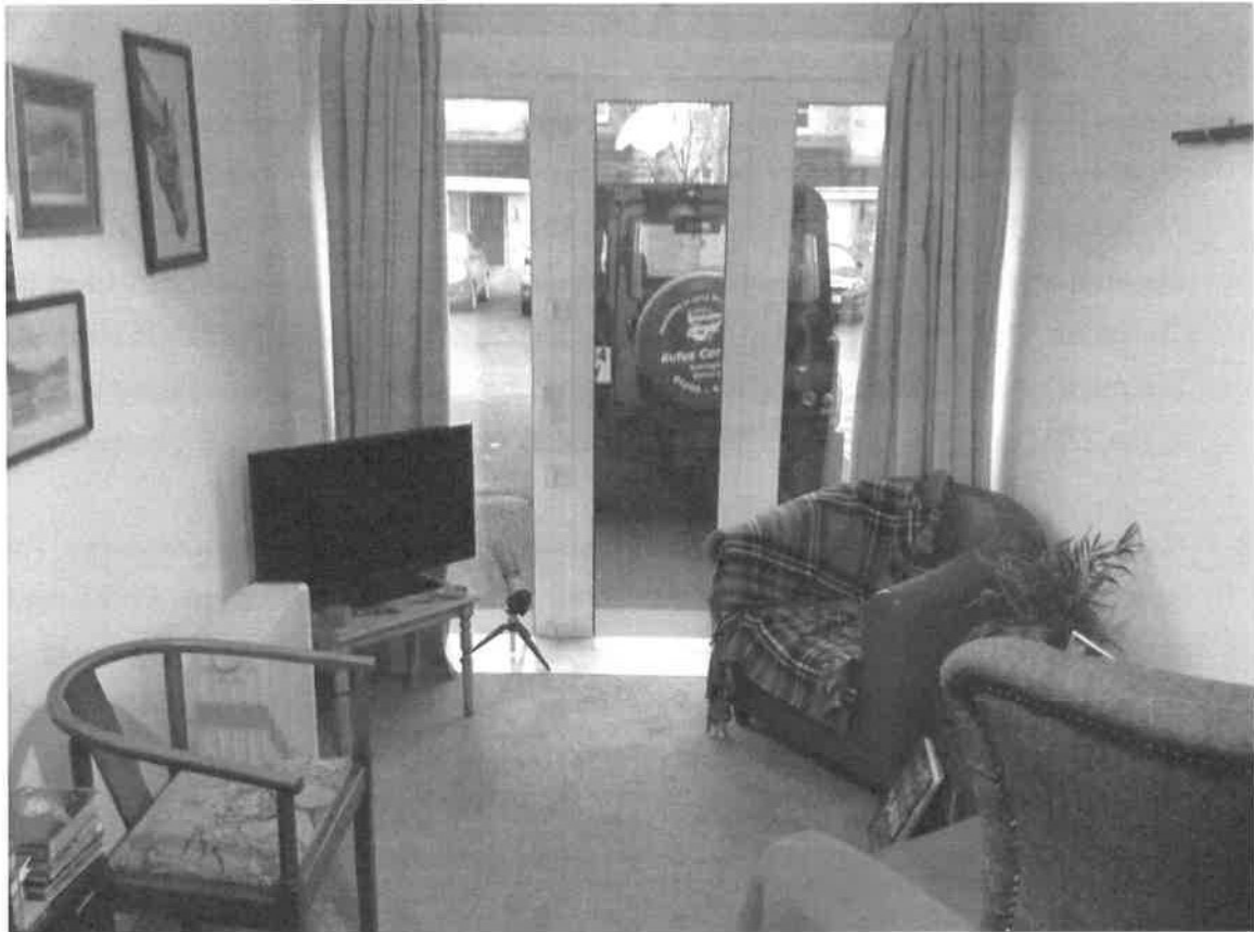
2 Interior of former garage now a sitting room at 32 Copperfield Close. The lower frame of the bi-fold doors is beneath floor level.
