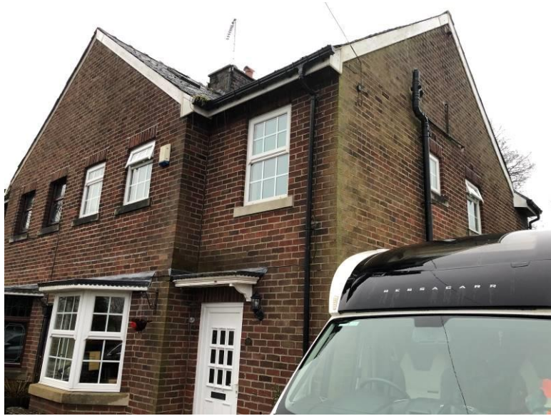
Plate 1: Front elevation of the property with occasional limited gaps at roof verges
