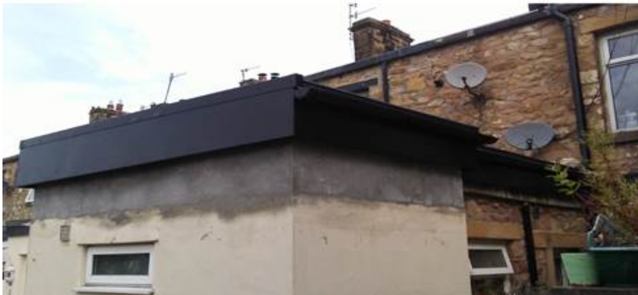
Fig 4: Photograph showing the current, later flat roof arrangement with external walls raised up to meet the continuous eaves level.
